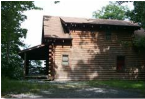
View of Outside of House
